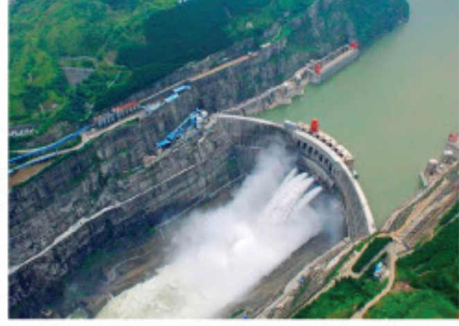
Xiluodu hydropower station
