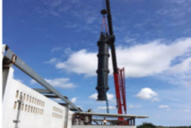
Texas flood control, USA
